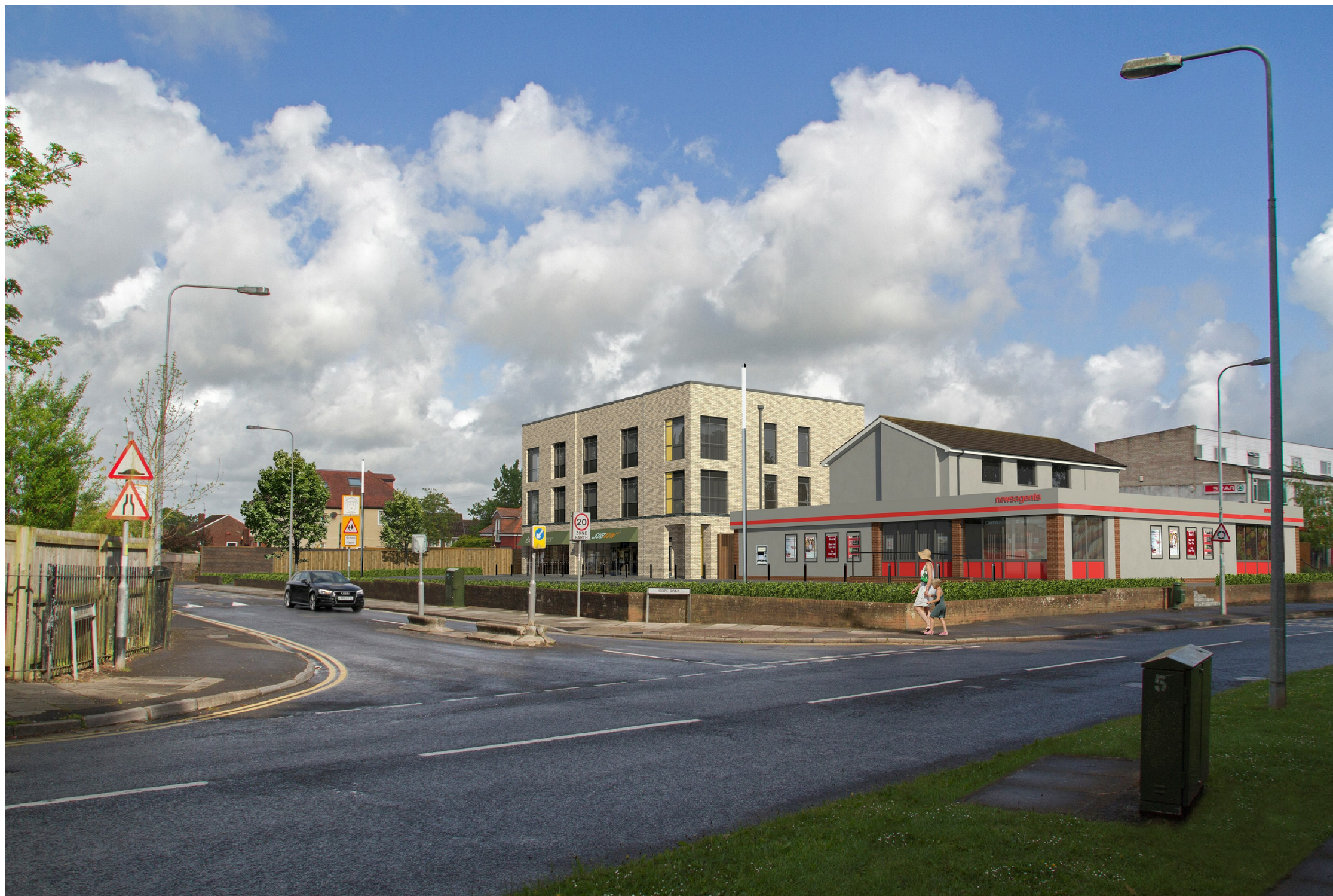
View from South East on Michaelston Road
